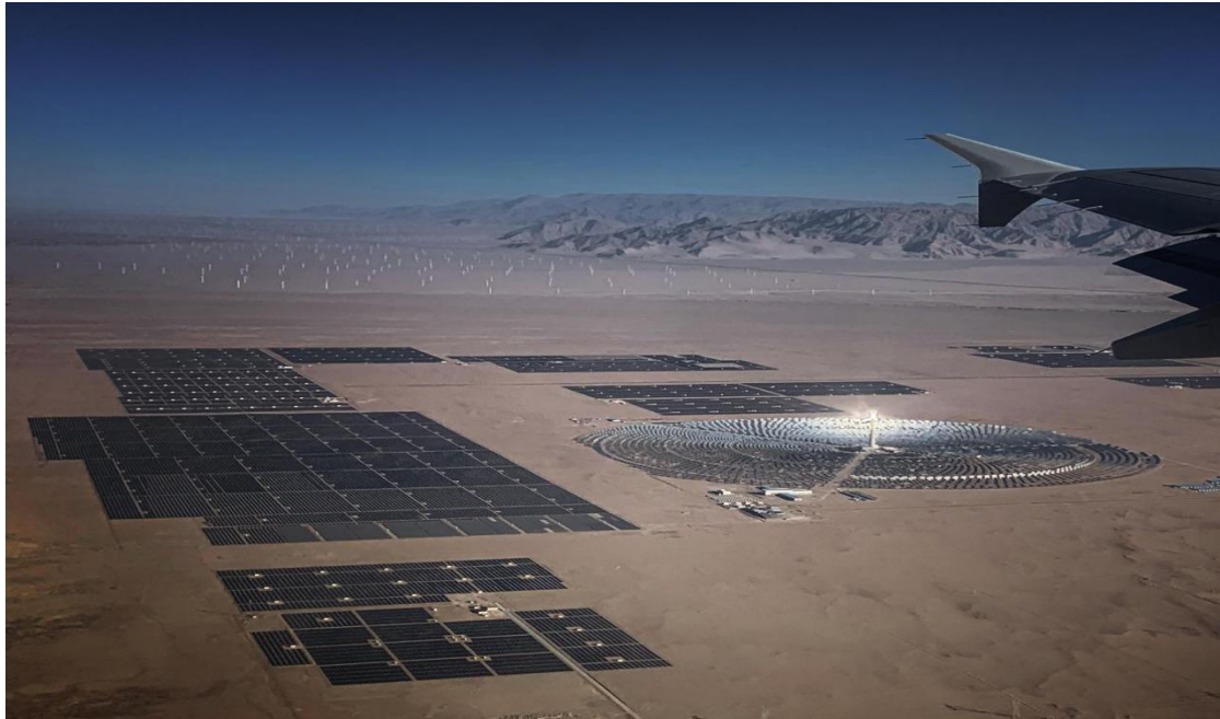
青海格尔木鲁能海西 50MW 光热电站 50MW Concentrated Solar Power Plant in Golmud, Qinghai Province
